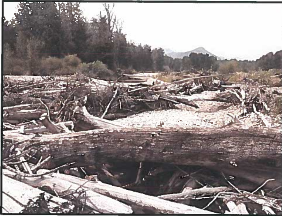
Figure 5. Photograph depicting large mid-channel log jams in the project area (view from the north).
